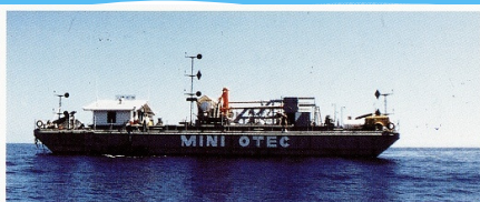
The first closed cycle Mini-OTEC plant to produce net power (15 kilowatts) at Keahole Point, Hawaii, in 1979
