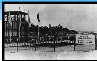
Nauru OTEC Project (1982~84)
